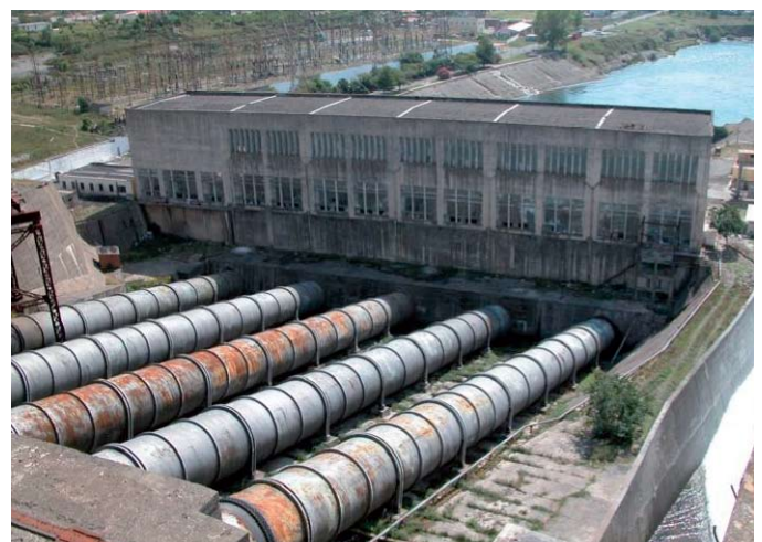
Below: Figure 3 – Deficiencies in hydromechanical equipment: Leakage of spillway gates (left) and corrosion of penstocks (right)
