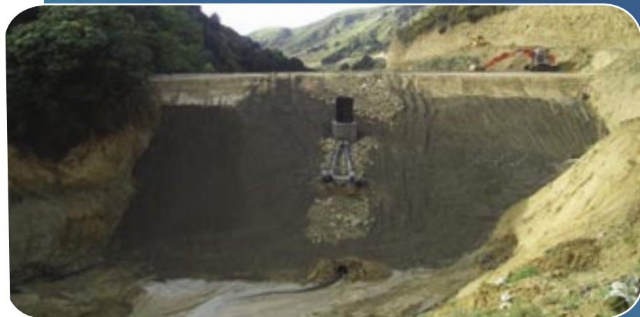
Front Cover Mangamahoe Dam Spillway May 2005
