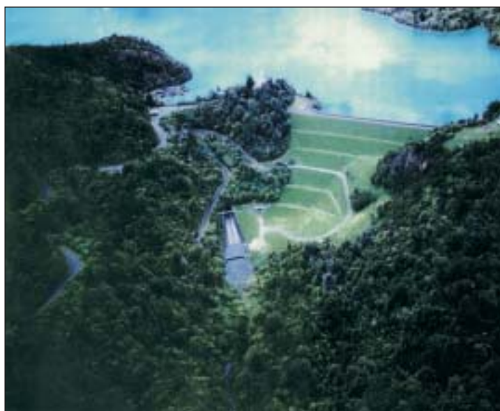
Figure 1. Cosseys Dam before works began.
