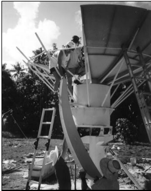
FIGURE 3. Installing petals on the Fakaofu antenna.
