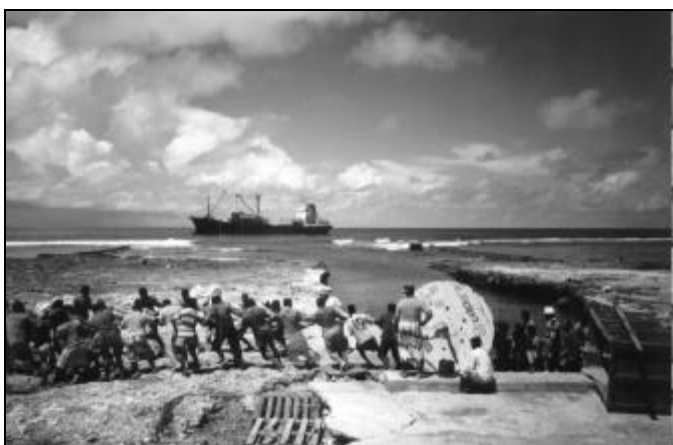
FIGURE 6. Unloading the 2.6 tonne armoured cable drum from a lighter, Fakaofu.
