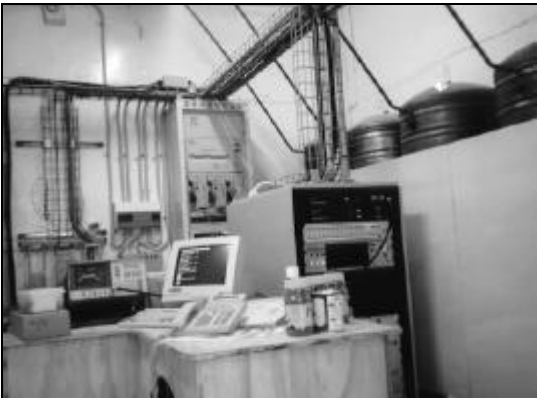
FIGURE 4. Fakaofu equipment room showing the STAR coolers on the right-hand wall.
