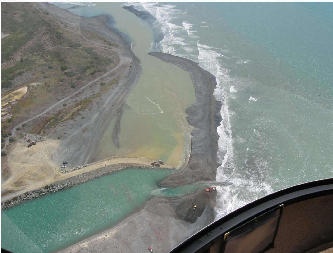
FIGURE 5: Wairau River mouth Jan 2009, cutting newmouth through bar, extending rock guide bank and cutting off old mouth.
