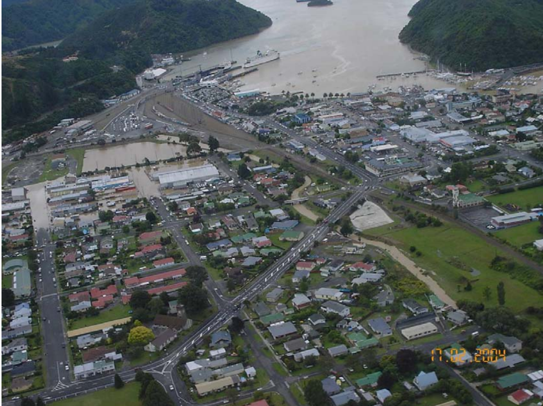
FIGURE 7: Picton February 2004, Industrial area flooded due to inadequate size of culvert under wharves
