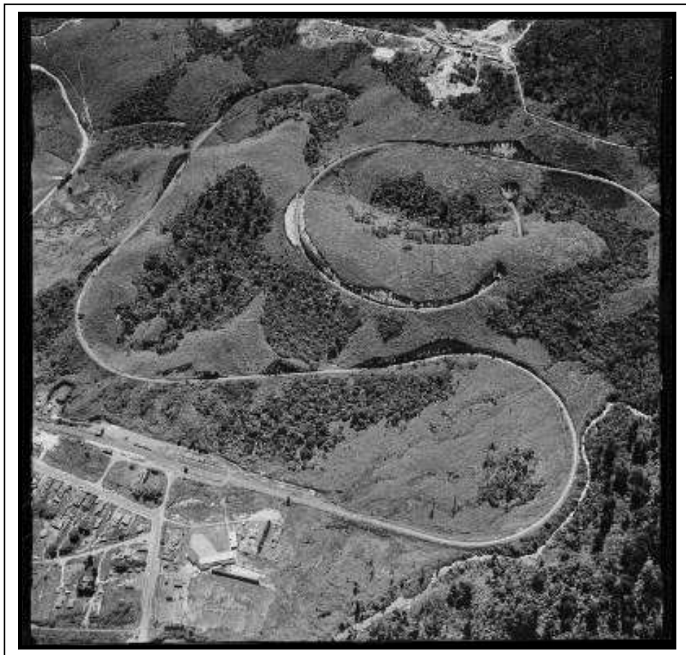
Aerial view of Raurimu Spiral on the Main Trunk railway line between Auckland and Wellington, with Raurimu township at the bottom left. Photograph taken 24 January 1957 by Whites Aviation. Alexander Turnbull Library (ATL), ID: WA-42886-F
