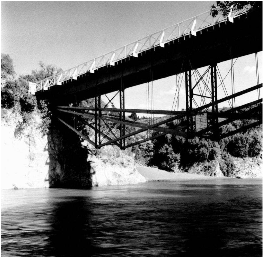
Figure 6: Rakaia Gorge Bridge, November 1997. Geoffrey Thornton Photographic Collection, IPENZ
