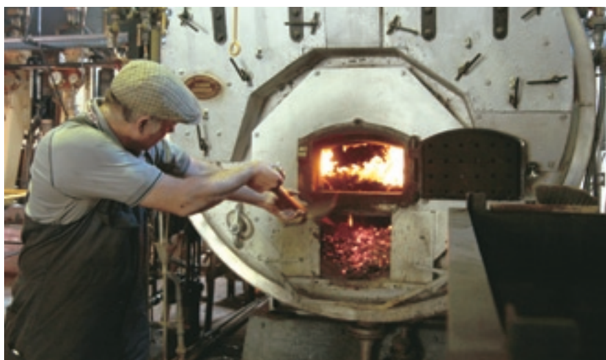
Stoking the boiler that will power the beam engine.
