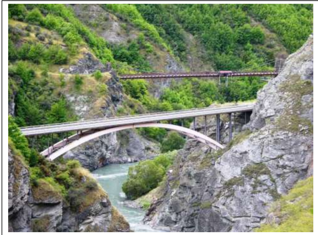
Figure 2: The 1963 highway bridge with Kawarau Gorge Suspension Bridge in the background, January 2006. Photograph courtesy of Lloyd Smith
