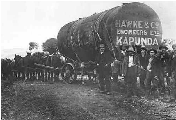
Figure 9: Boiler transport to Talisker mine [SLSA B 17641]
