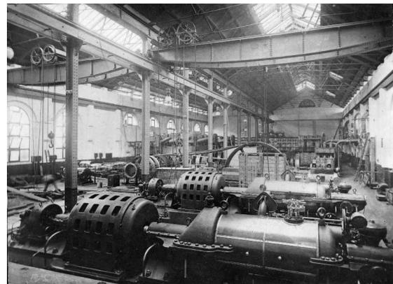
*Figure 5 SSPS Engine Room c1908 showing T/As*
