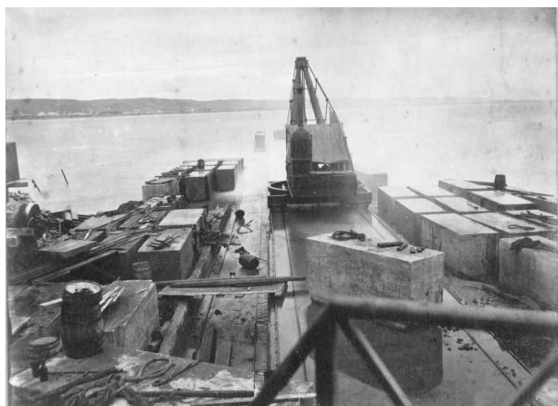
Figure 2: The steam crane 'Moa' working in deteriorating weather conditions. – North Otago Museum 4058
