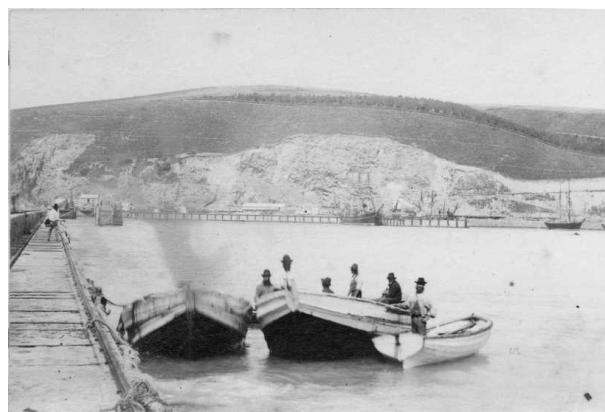
Figure 3: Early in 1883. A couple of surf boats are at the end of the breakwater and a wooden caisson is being towed along Macandrew Wharf to be sunk to form part of the breakwater tip. Another caisson is taking shape behind the Cross Wharf in the background. – North Otago Museum 4050
