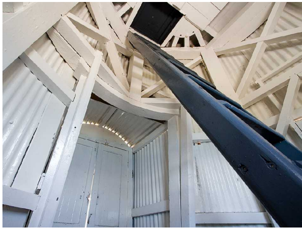
Figure 6. Interior of Goods Island lighthouse
