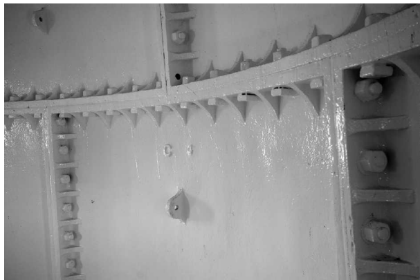
Figure 2. The cast iron plates of the Bustard Head lighthouse tower
