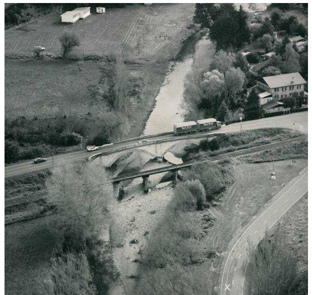
Figure 7. The northern Waianakarua bridge.
