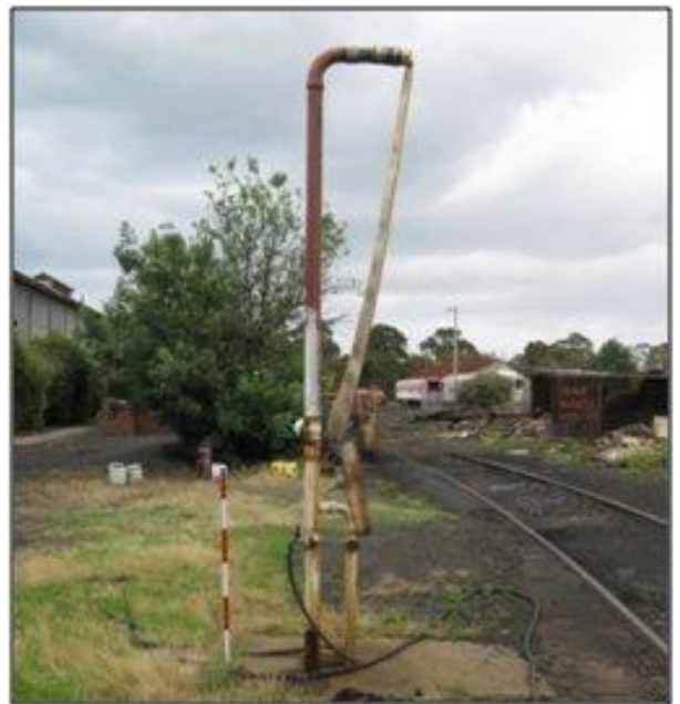
Figure 3-3 Area A view south, standpipe ca 1933 and active line in limited use (Holmes P. 2008, ‘Newport Stabling Yards Baseline Historical Assessment’, Report, Department of Transport, Melbourne)
