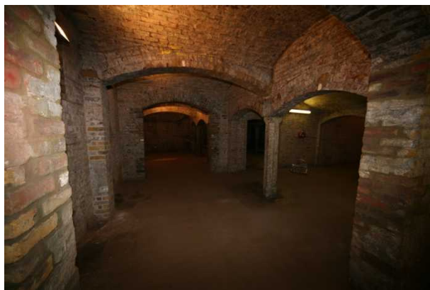
Figure 13 General view of Clerkenwell vaults
