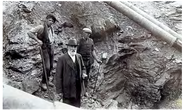
Figure 11. John Ewing (front) on site
