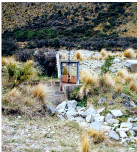
Figure 4. Ten Chain Creek Bywash and control on Mt Ida Race in top section
