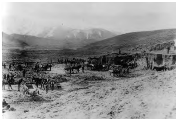
Figure 2. West Eweburn Dam construction 1898?
