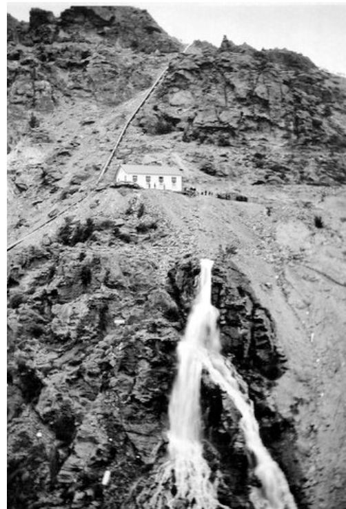
Figure 17. Original Teviot (George) power station
