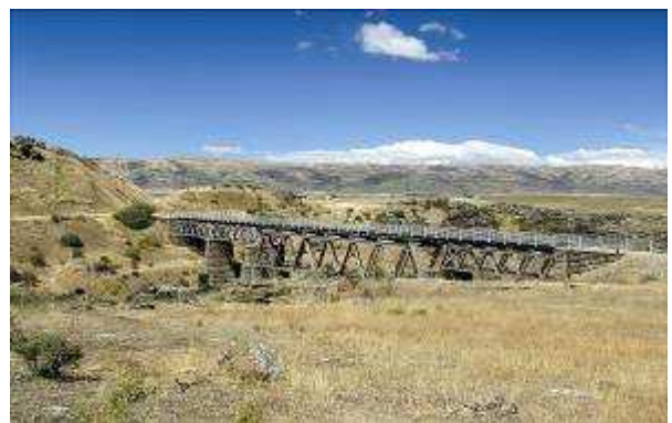
Figure 10. Poolburn Viaduct with Dunstan Mountains beyond.
