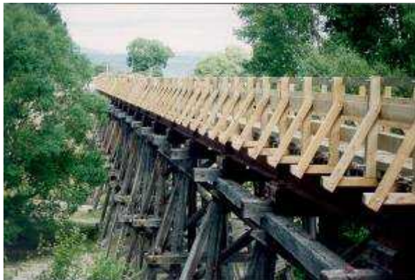
Figure 12. Muttontown Viaduct near Clyde showing raker bracing.
