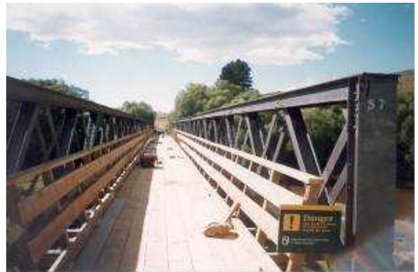
Figure 9. Waipiata Bridge being re-decked for cyclists and walkers.
