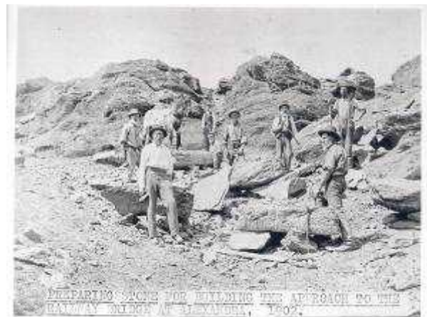
Figure 3. Stonemasons at work cutting stone for another Otago Central Railway bridge - Hocken Library
