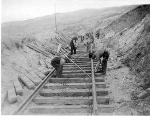
Figure 5. Workers laying tracks on the Otago Central Railway - Hocken Library.
