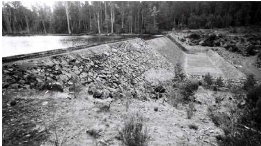
Figure 3. Hydro Tasmania Dam with stone walling of heritage value.
