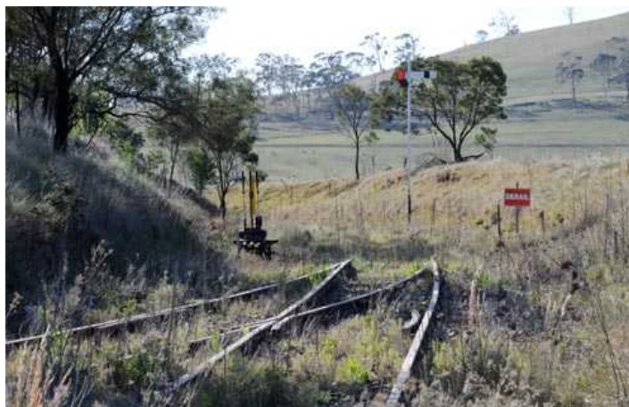
Figure 8. Dumaresq Railway Yard with abandoned infrastructure.
