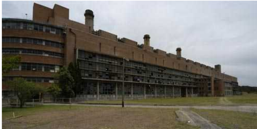
Figure 6. Wangi Wangi Power Station
