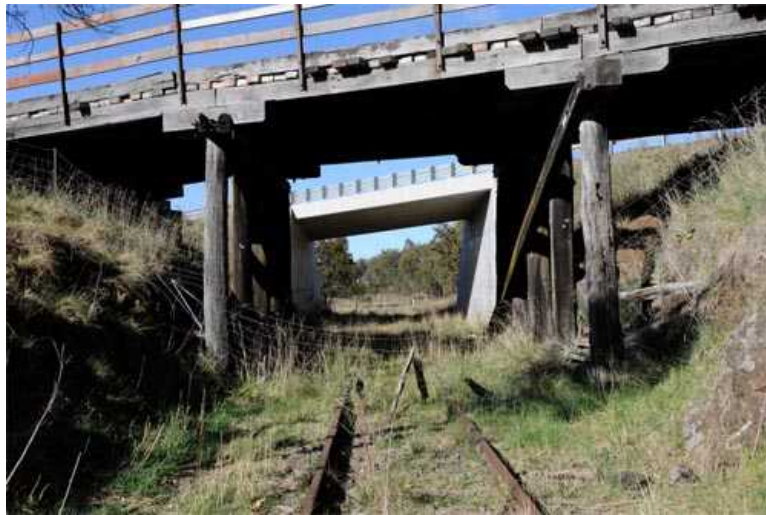
Figure 9. Dumaresq road bridges, old and abandoned and new beyond.
