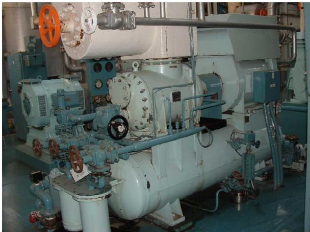
Figure 10: A relatively early model twin screw compressor
