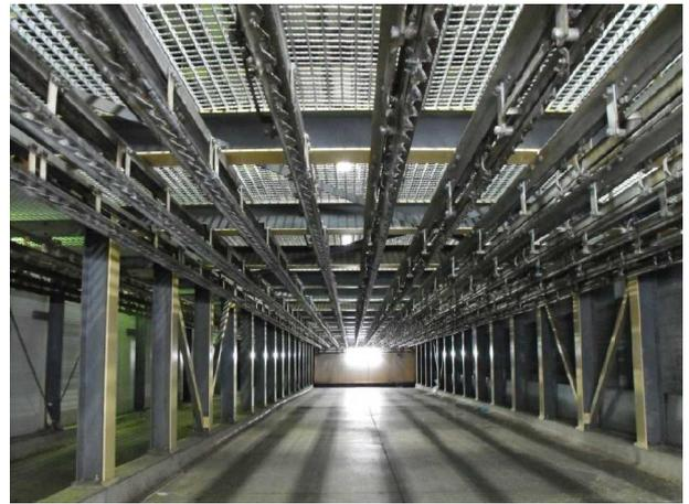
Figure 4: Typical modern air-blast carcass freezer
