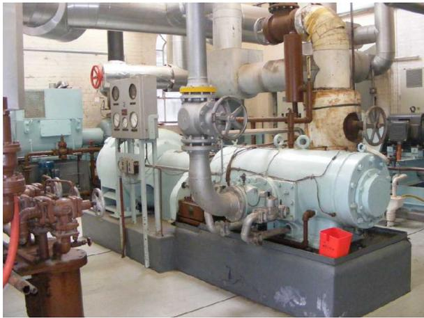
Figure 9: A typical rotary vane booster compressor.
