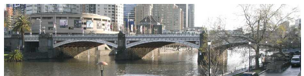
Figure 6. Princes Bridge Today
