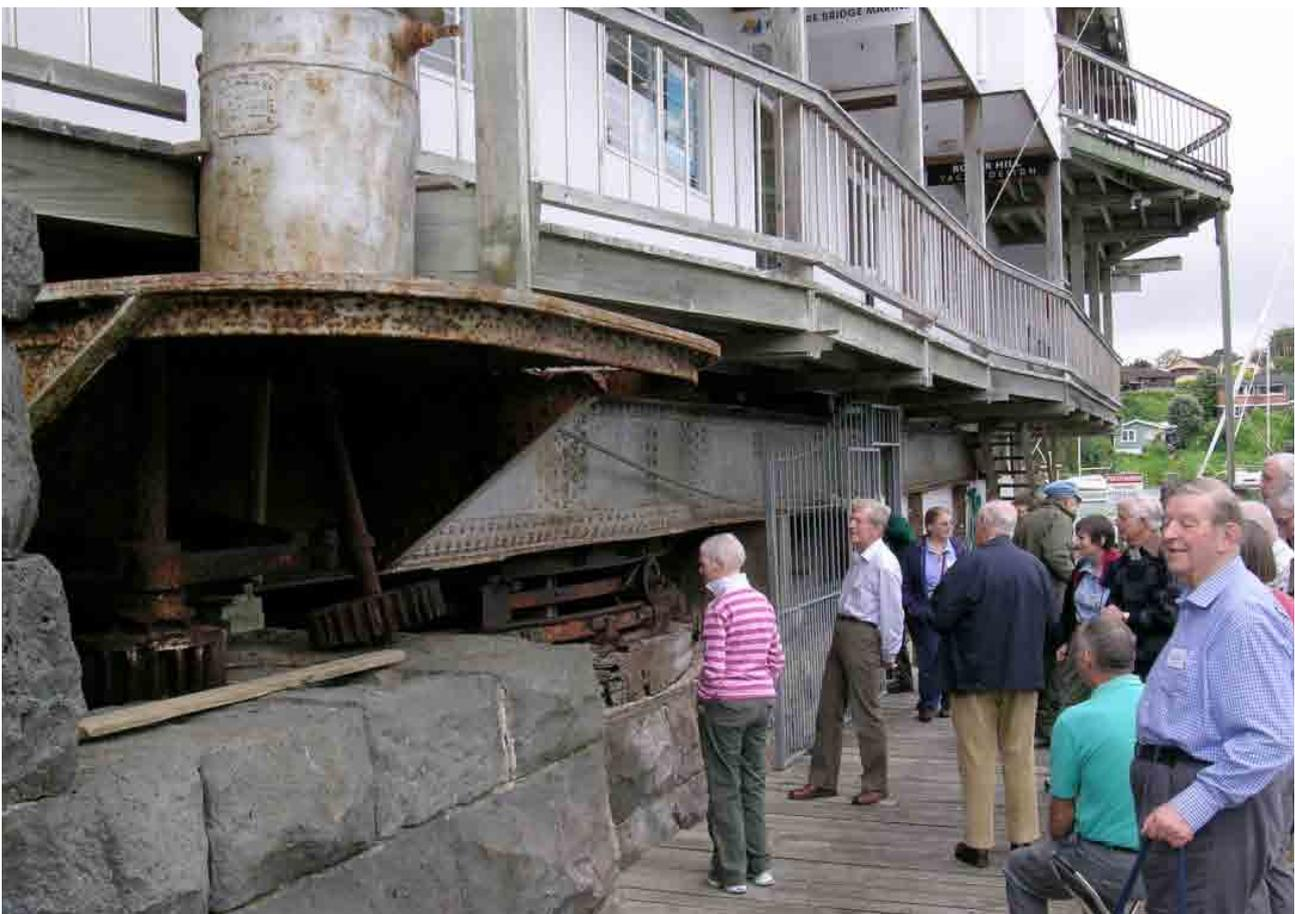
*The Tamaki River Bridge, in Panmure Auckland, was built in 1864–65 with a 40-foot swing span, seen here under a ships' chandlery store. The cylinder on the left is the hand-operated winch originally used to turn the swing span which rotated on a circular rail.*
